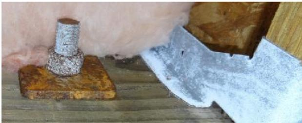
**Figure 8-50** Six-year old installation in a mechanically vented crawlspace, where air circulation was provided by a fan to provide reliable ventilation. It would take a fairly long time—maybe decades—for this bolt to corrode to the point it lost significant strength. Nails are a different matter; see below.
