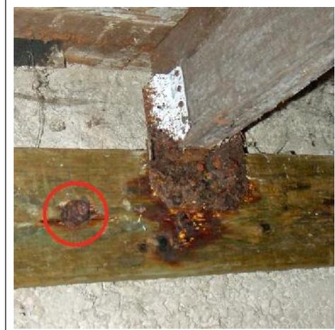
**Figure 8-45** Most wood now sold to resist decay also attacks steel connectors. The red circle shows a rusted concrete anchor. At center is an H10 (compare to Figure 6-34). This installation was about 10 years old.
