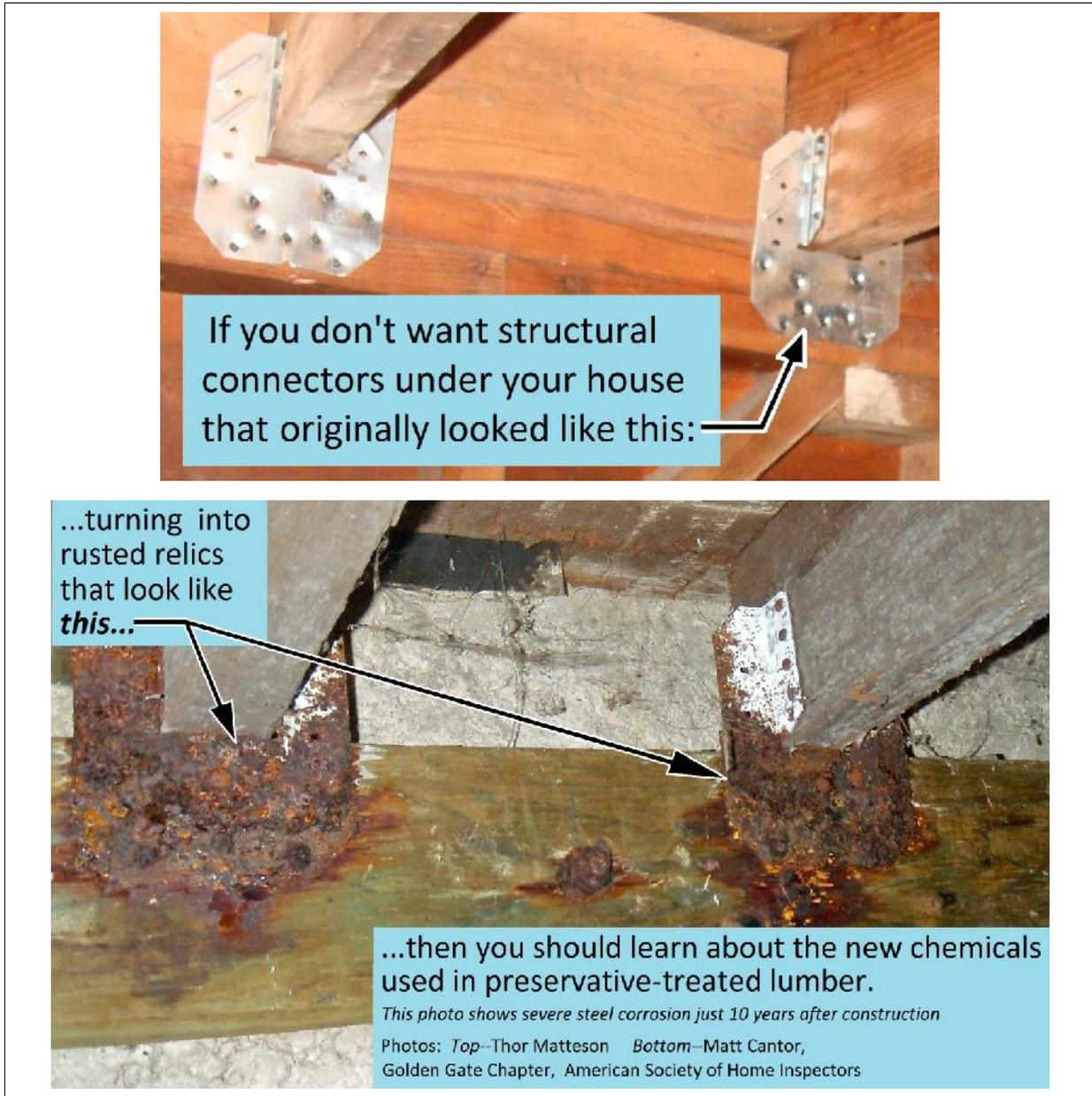
This handout is part of an upcoming book on earthquake retrofits by Thor Matteson, Structural Engineer. Mr. Matteson has been concerned with fastener corrosion since 2004, when the wood-treating industry began using new preservative formulations that aggressively attack steel hardware. Mr. Matteson is the author of “*Wood-Framed Shear Wall Construction—an Illustrated Guide*”
