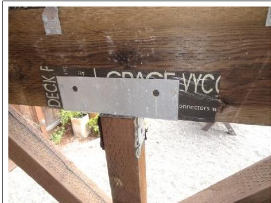
**Figure 8-54** PT lumber separated from a sheet metal connector with a self-adhered membrane. The nails still penetrate the PT lumber. This method may delay corrosion in the connector, but the membrane does not offer any improved protection for the nails.
