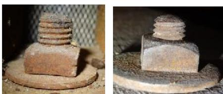
**Figure 8-48** Bolts shown above were installed before PT chemical reformulation and show minimal corrosion. *Left: In a CCA mudsill, approx. 35 years old; Right: In a redwood mudsill, approximately 80 years old.*
