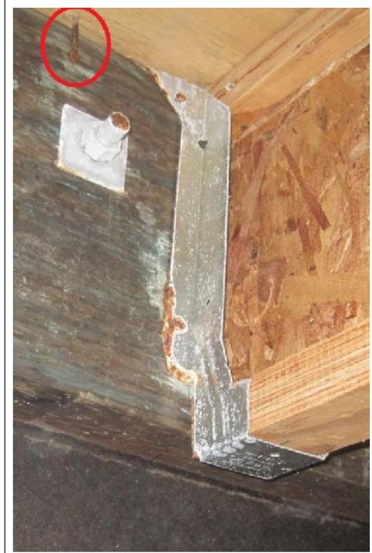
**Figure 8-49** This installation was four years old when photographed. Note the red circle at the top of the picture, which shows a rusted nail that is just barely touching the PT ledger.
