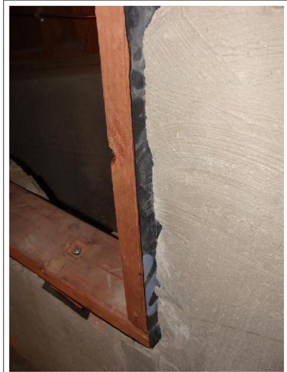
**Figure 8-56 Untreated lumber shown here is protected from moisture wicking through the concrete foundation wall by “peel-and-stick” membrane (also called self-adhered flashing, commonly used to waterproof around window and door openings).**
