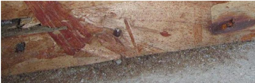
**Figure 8-51** Rusty edge nailing of a shear panel, approximately five years after construction. Contractors have reported almost total corrosion of nails in just a few years. Photo by Skip Walker, Silicon Valley ASHI/CREIA
