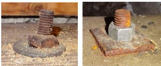
**Figure 8-53** Anchor bolt on left is from original 90-year-old construction. Anchor on right was installed in PT lumber for an eight-year old remodel in the same crawlspace. The anchor in the PT material looks worse than the older one. Photos: Justin Brodowski
